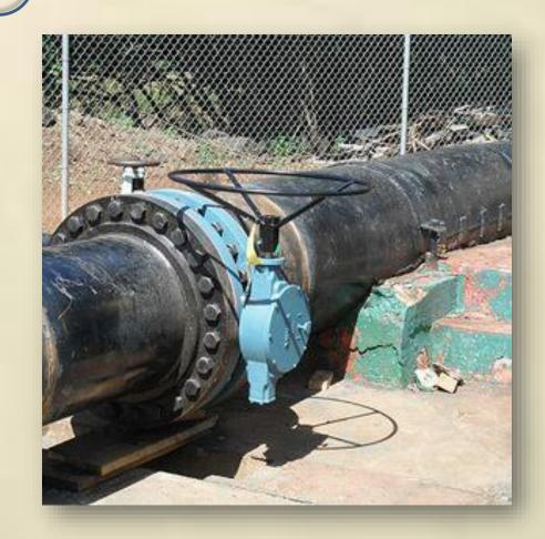
We introduce ourselves as the leading manufacturer and supplier of **Butterfly Valves** in India. The offered butterfly valve is a Quarter-turn rotational valve which is used to stop, start and regulate the flow, that is easy and fast to open. The handle of the valve can be rotated to 90° rotation and provides a complete opening or closure of the valve.
